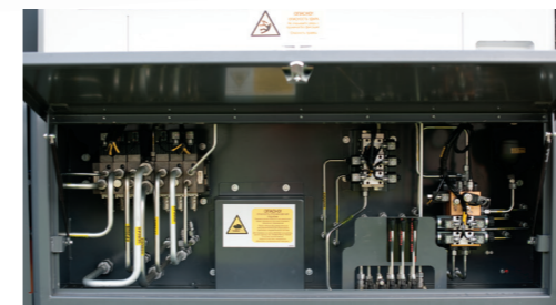
Steel pipework for better heat dissipation
